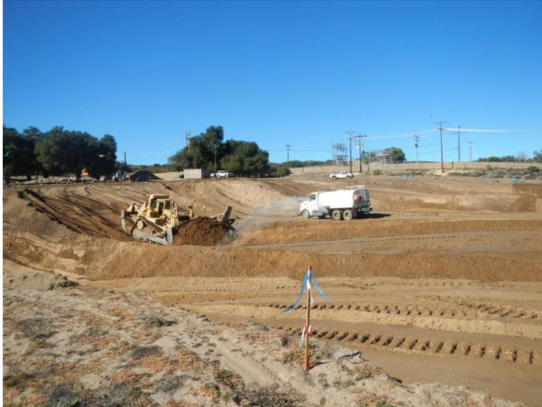
**Photo 1:** Water trucks are utilized on a regular basis to minimize fugitive dust emissions in accordance with MM-BIO-4A and the Dust Control Plan at the Boulevard Substation Rebuild site.
