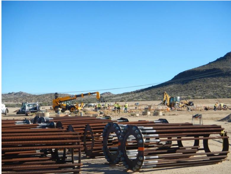
**Photo 3:** Construction crews completing concrete foundations for the control and maintenance shelters at the 138/230 kV ECO Substation pad.
