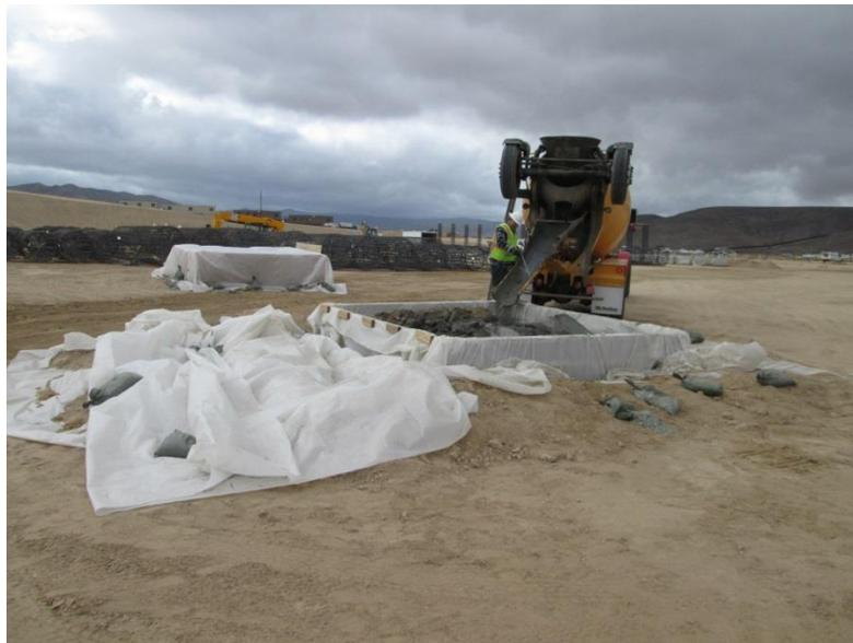
**Photo 4:** A concrete washout basin is being utilized for washing out concrete trucks following foundations pours at the 138/230 kV pad site in accordance with the SWPPP and MM-HYD-1.
